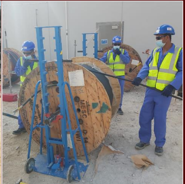
Duqm Refinery EPC-2 Al Ansari Projects
