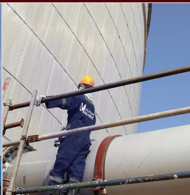
Duqm Refinery - Testing & Inspection Works
