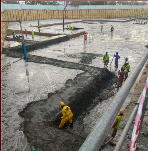
Civil Works, Philips Pharmaceutical
