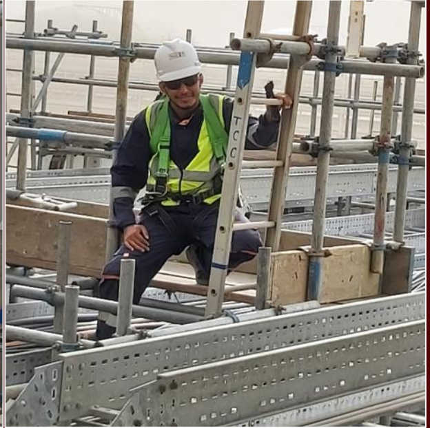
Duqm Refinery EOC2 Al Ansari Projects
