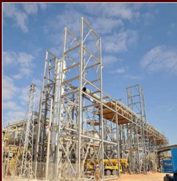
Duqm Refinery - Fabrication Work
