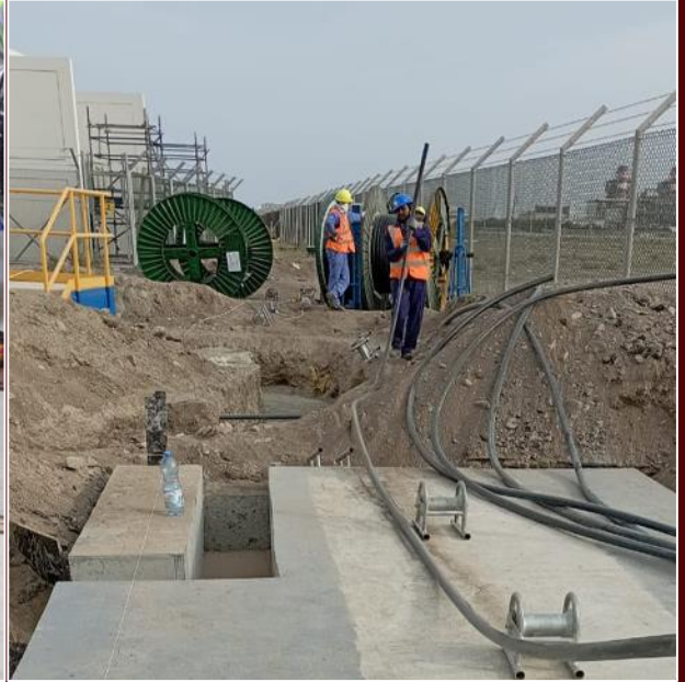
Majis Industrial Services, Sohar Port Project
